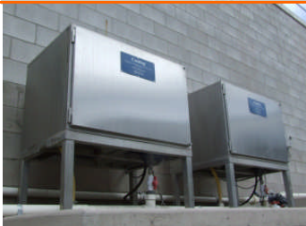
Typical Coolfog pump modules S/S boxes
